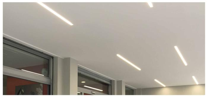
Decorated anodised aluminium lamp complete with brushed or microprismatic diffuser and high-brightness LED source with a high Lumen/Watt ratio. Suitable for primary residential, retail, large-space and general lighting. The interlocking profile mechanism allows for easy maintenance. Flush-mounted installation onto plasterboard or brick, also supplied with non-returnable cover for plastering.
